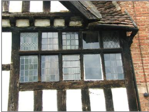
Transom and mullion casement windows (left) and a projecting window with supporting brackets (right) on timber framed buildings
