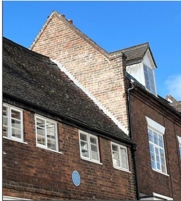
Lead flashing stepped with the mortar courses
