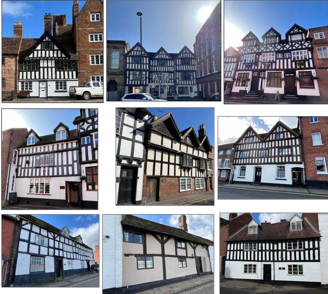
Variations of timber framing in the Conservation Area
