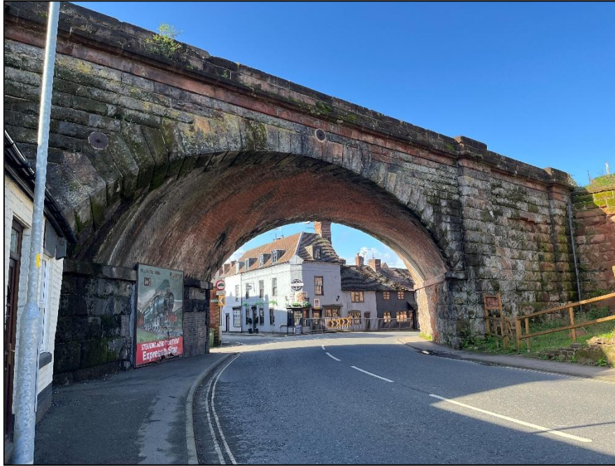
Viaduct over the Kidderminster Road
