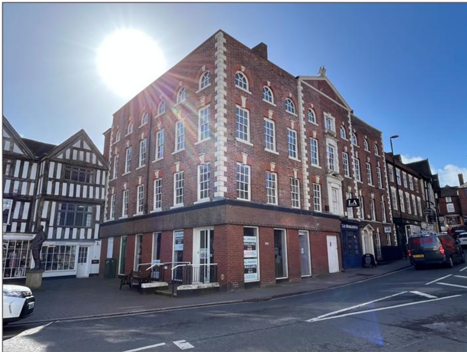
Unsympathetic alterations to the ground floor of former HSBC in Load Street
