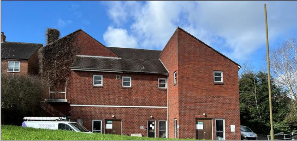
Telephone Exchange, Dowles Road
