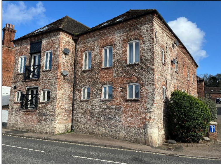
Former warehouse (now flats) adjoining Stourport Road in Wribbenhall
