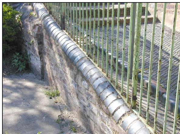
Traditional semi-circular coping to the top of a wall
