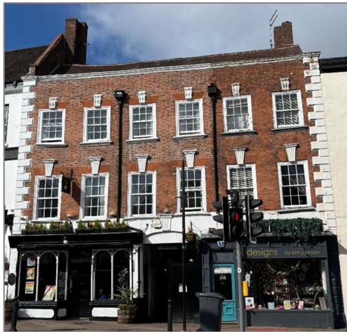
A selection of Georgian sash windows found within the Area, with gauged headers (top left) gauged headers & keystones (bottom), and in the Venetian style with applied headers (top right)
