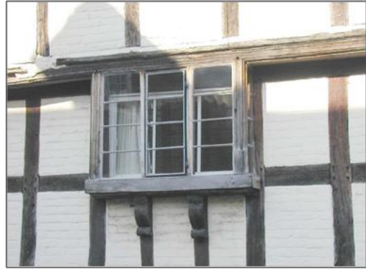
Transom and mullion casement windows (left) and a projecting window with supporting brackets (right) on timber framed buildings
