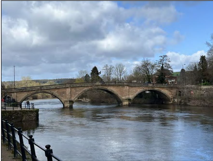
Central Bridge, designed by Thomas Telford
