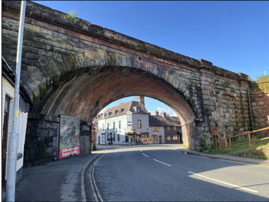
Viaduct over the Kidderminster Road
