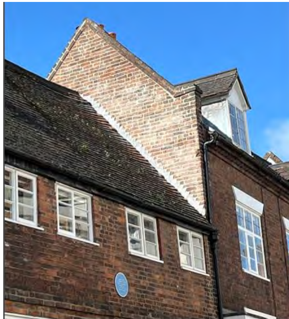
Lead flashing stepped with the mortar courses
