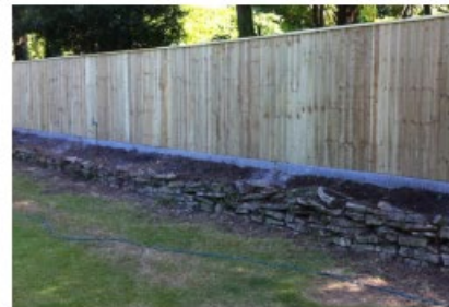
Timber closeboard fence on the top of the existing wall to the north.
