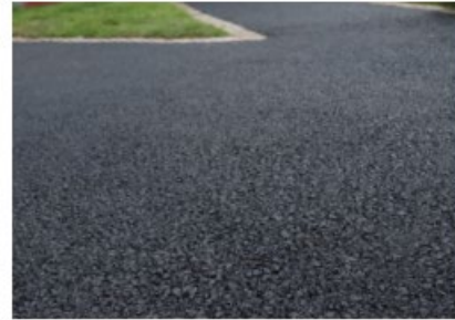
Asphalt to vehicular entrance.
